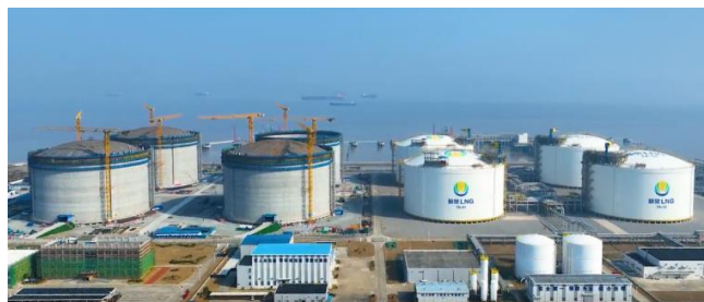
Four new tanks successfully launched in Zhoushan Terminal Phase III, marked by the operation of gas pressure lifting
