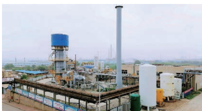
Natural Gas Hydrogen Production Project in Liaoning Province
