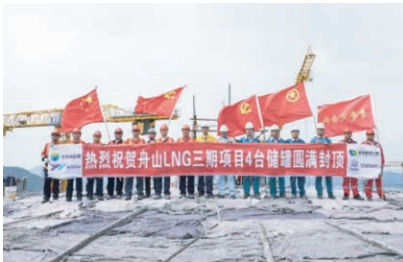
Four new storage tanks of Zhoushan LNG terminal successfully capped
