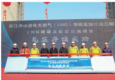
Successful gas pressure lifting for Zhoushan Terminal Phase III project
