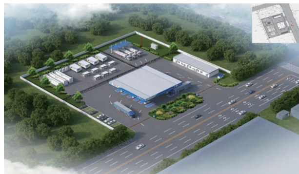
The Guanghui Green Power and Hydrogen Production and Integration Demonstration Project
