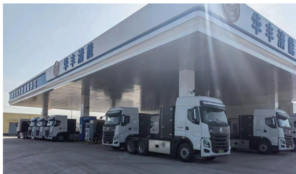
Huafeng Hydrogenation Integrated Energy Service Project
