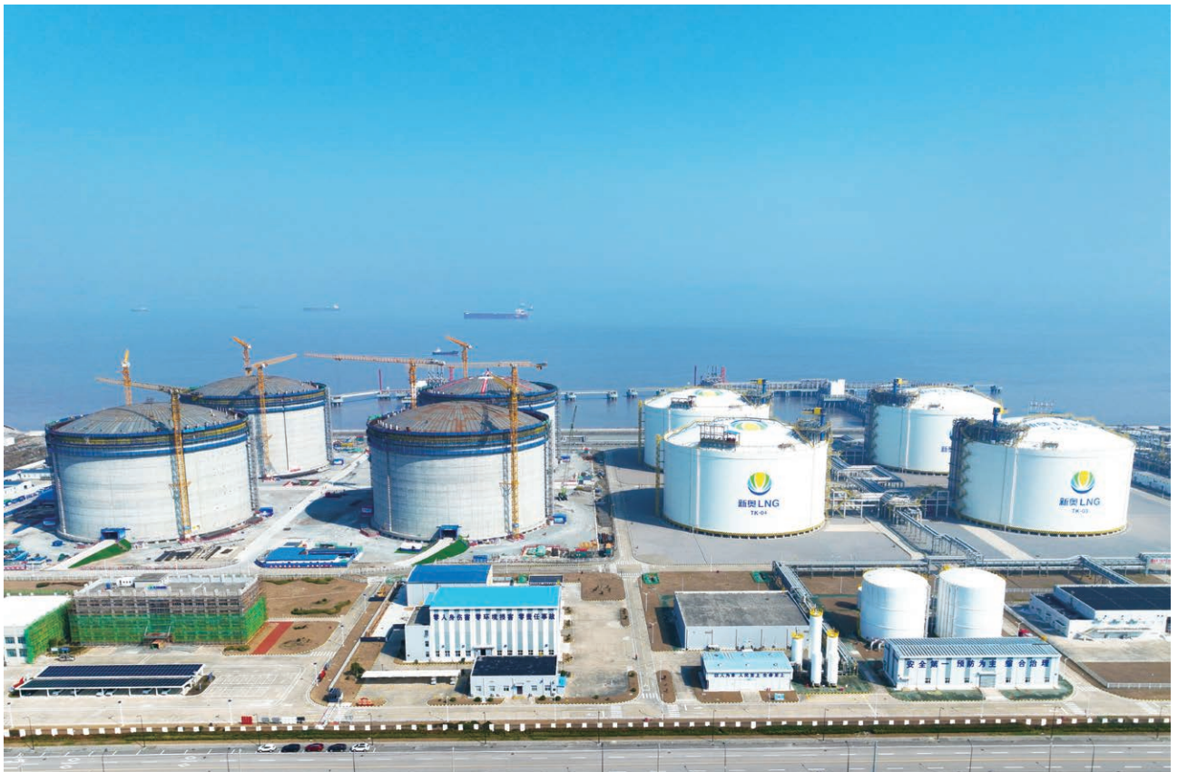
Zhoushan Terminal Phase III project
